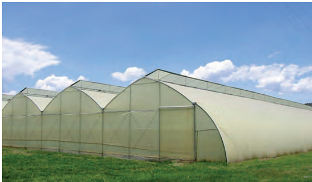
Fig. 7.4 Typical naturally ventilated polyhouse (NVPH)
